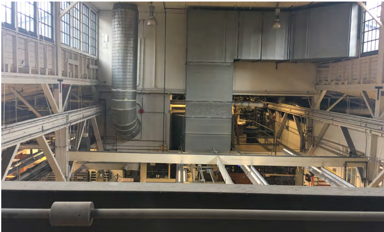
Figure 50. Main volume looking north from the mezzanine. The solid wall in the background is the original location of the wall separating the second floor from this area.
