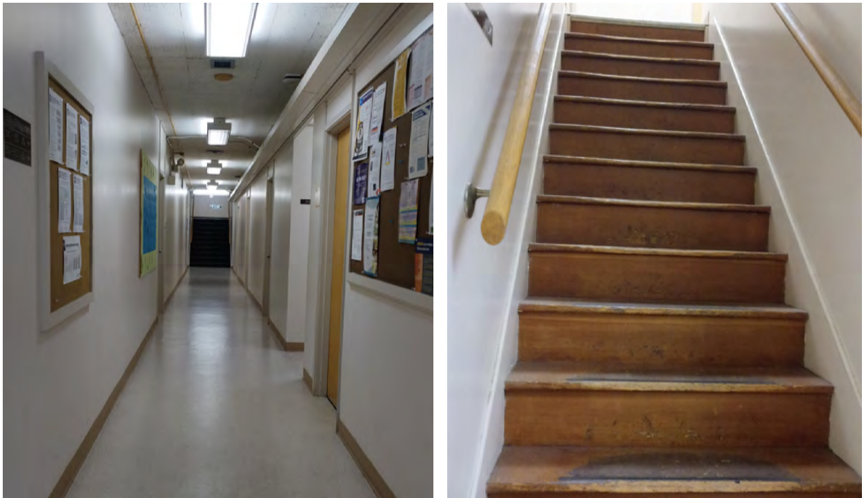
Figure 65. Second story, north end, typical corridor detail (above left), and typical stairway to third floor (above right).
