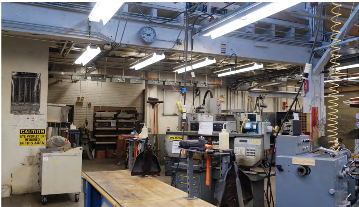
Figure 55. Main volume, looking south, the mezzanine level is visible along the top of the photograph.
