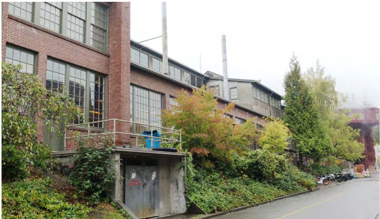
Figure 45. East facade, looking northwest.
