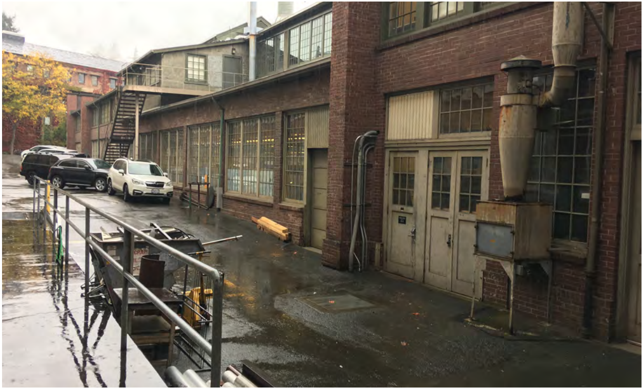
Figure 34. West facade looking north.
