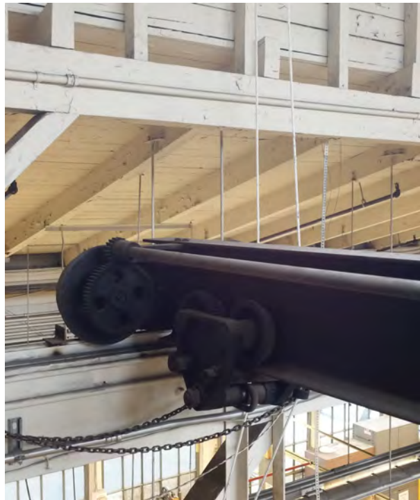
Figure 53. Main volume crane details from the mezzanine level.
