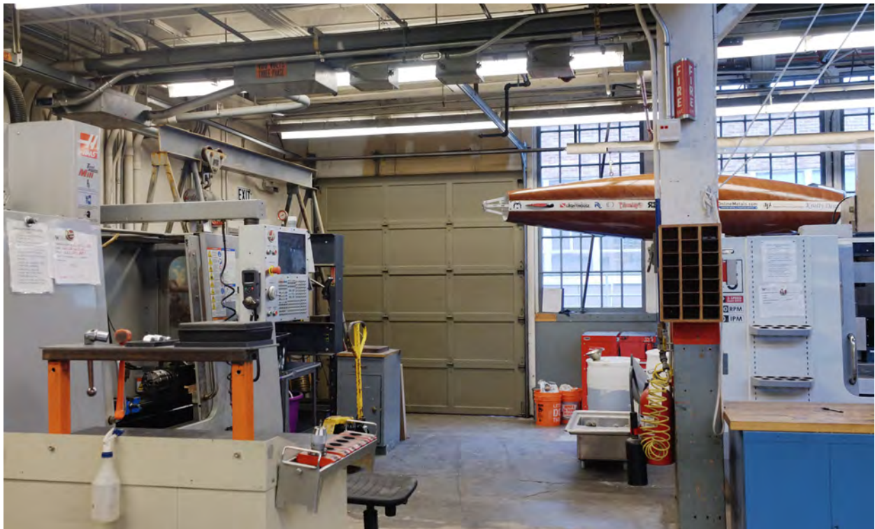
Figure 54. Main volume, looking west towards the garage door entrance.
