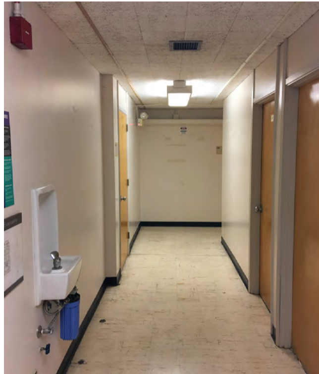
Figure 68. Third floor, north end, typical corridor configuration.
