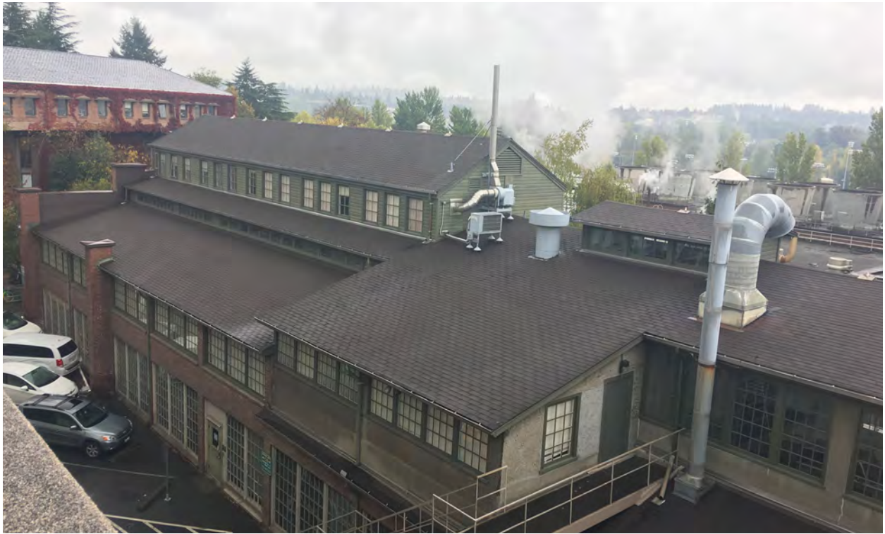
Figure 36. Looking northeast from the roof of the MEB.
