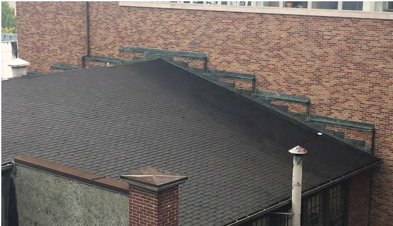
Figure 39. South end wall connection with MEB detail.
